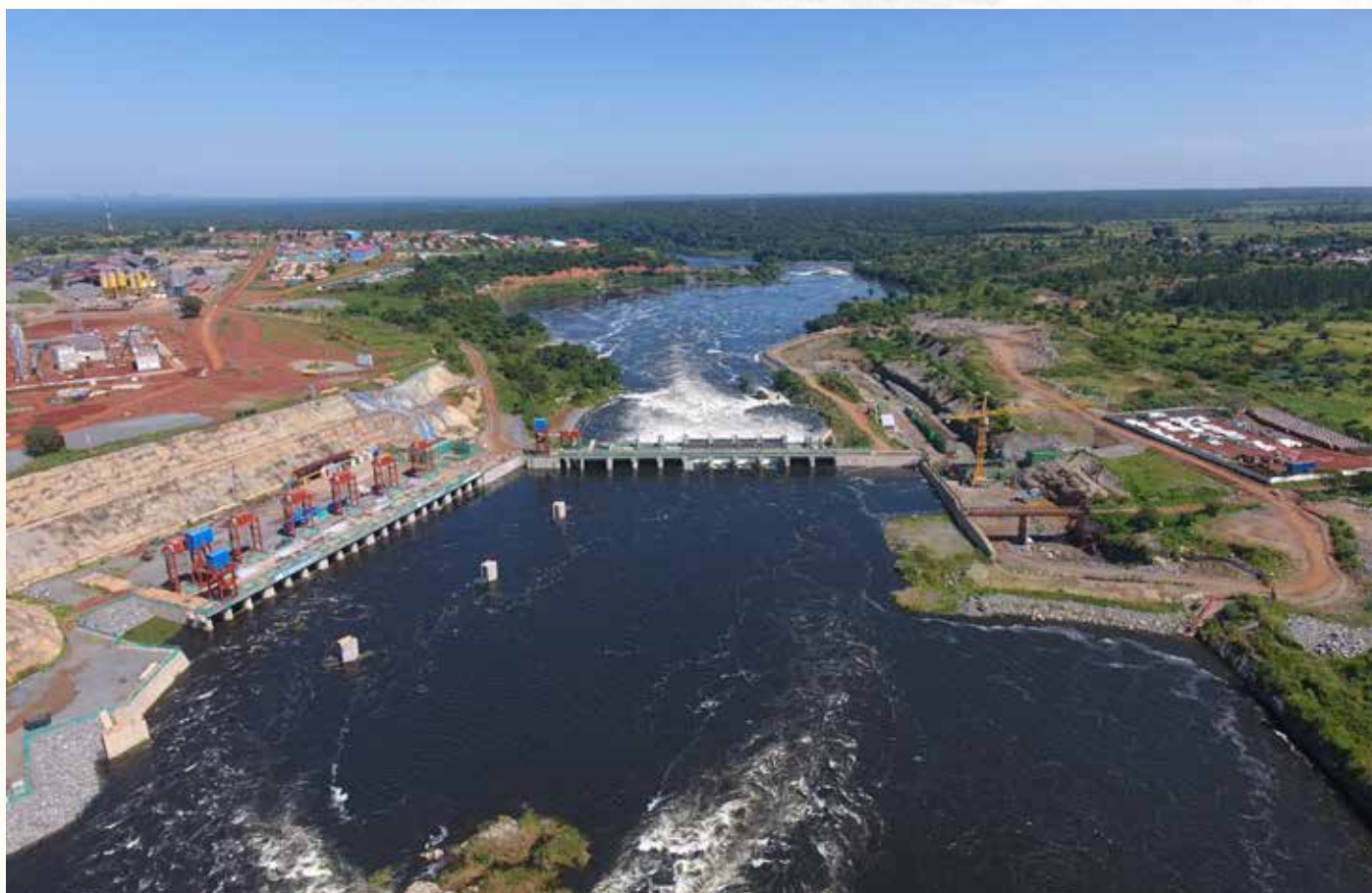
Once Commissioned, the 600 MW Karuma Hydropower Project is expected to further boost Uganda's Installed Generation Capacity.
